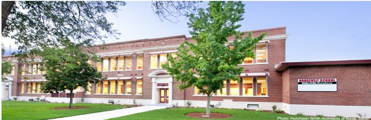
Photo: Hutchison Smith Architects of Boise, Idaho
