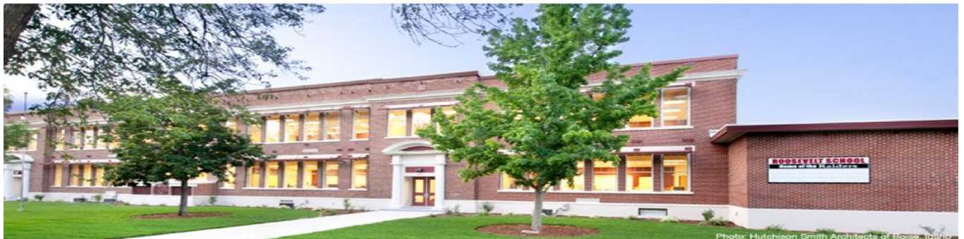
Photo: Hutchison Smith Architects of Boise, Idaho
