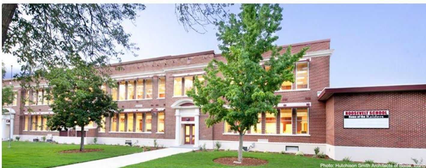
Photo: Hutchison Smith Architects of Boise, Idaho
