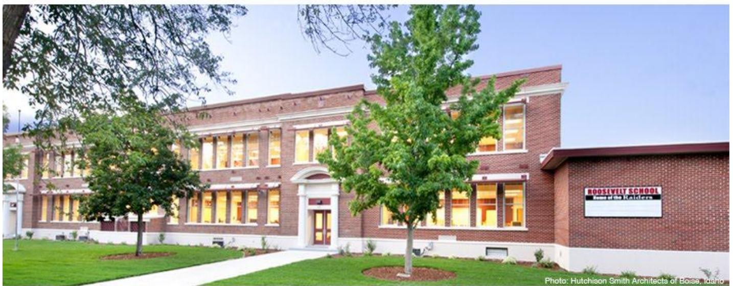
Photo: Hutchison Smith Architects of Boise, Idaho
